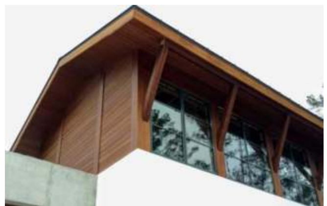
Engineered bamboo products used as rain screen and structural supports for the overhang (Source: Sullivan 2018)
