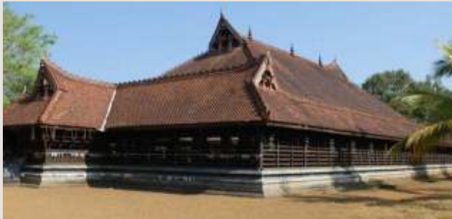
A Traditional Mass Timber South Indian Koothambalam (Sanskrit Theatre) Archeological Heritage Structure
